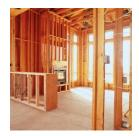
Build your walls using 2 X 4 or 2 X 6 inch studs and ceiling joists following the guidelines of local and state codes in your area. The thicker the walls the more insulation you can fit in. Try to use 6" studs on all exterior walls, if possible.
